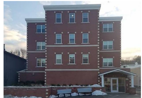
Nyack Point Apartments. (Courtesy Community Preservation Corporation)
